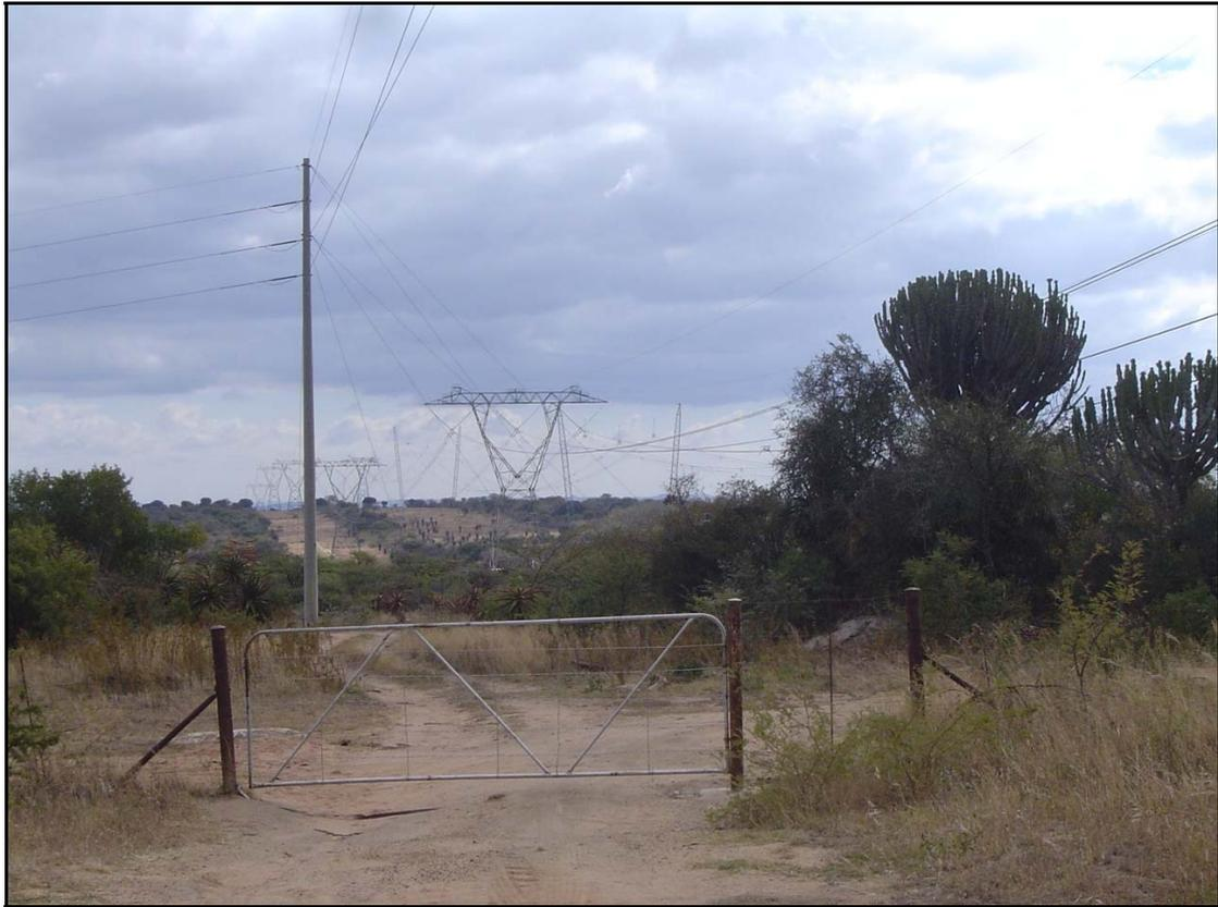
**Figure 9:** Existing Matimba-Witkop 400kV transmission lines (Note: The vegetation cover is removed underneath the power lines).
